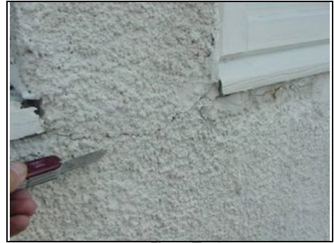
Hairline cracking to render
