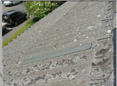
Asbestos roof
