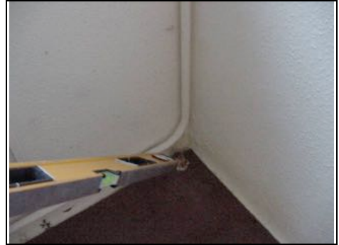
Kitchen cut off pipework
