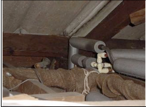
Unlagged pipework
