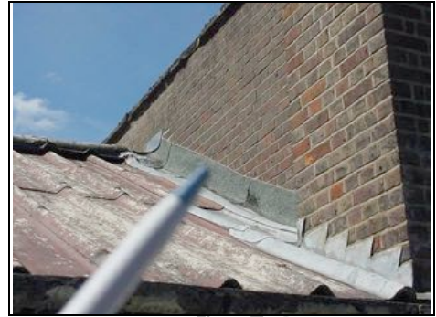
Poorly repaired flashing on adjoining property allowing dampness into your property
