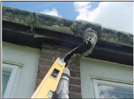
Asbestos gutters and downpipes in poor condition
