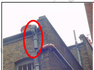
Redundant pipe
