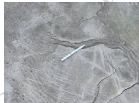
Cracking to asphalt
