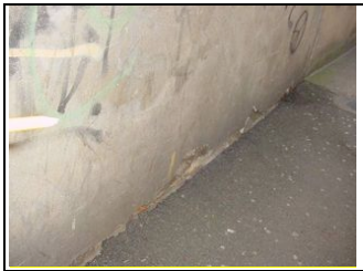
High external ground level to internal ground level
