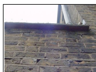
Flemish Bond Brickwork
