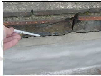
Gap where asphalt meets parapet wall.
