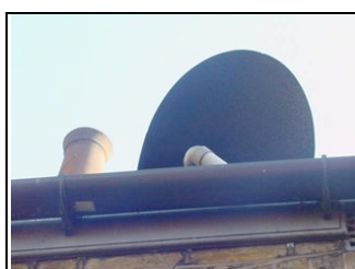
Waste pipes going into rainwater pipes XXXX
