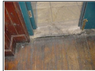
Ground level outside similar to ground level inside damp can therefore occur
