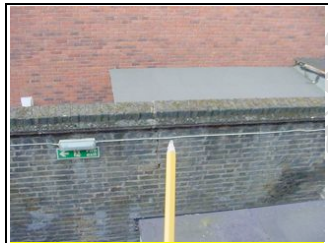
Cracking to rear boundary wall
