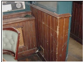
Damage to cladding
