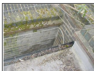
Gutter full of debris
