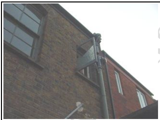
Broken window General staining to rear brickwork
