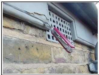
Rot to fascia and soffit
