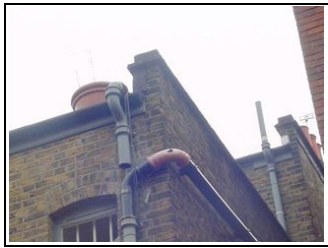
Redundant soil and vent pipe
