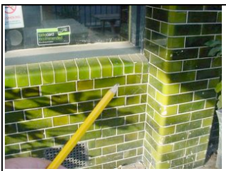
Close up of cracking
