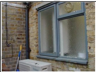
Casement window needs repair and re-decoration
