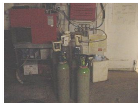
Gas cylinders not chained
