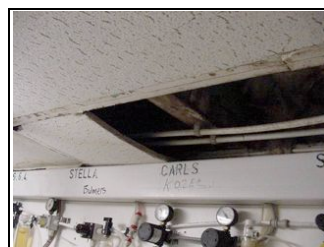
Missing ceiling panel
