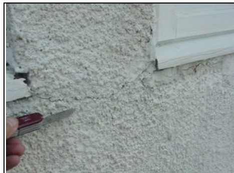
Hairline cracking to render
