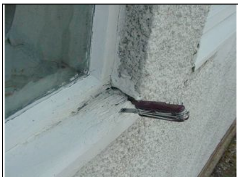
Rear window knife test
