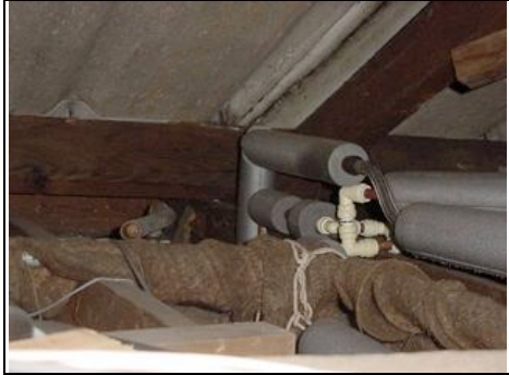
Unlagged pipework
