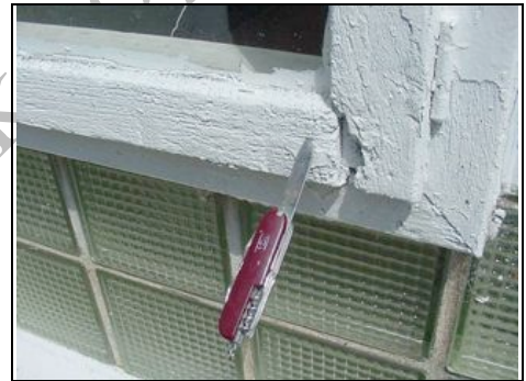
Knife test to timber window
