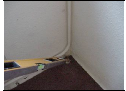
Kitchen cut off pipework
