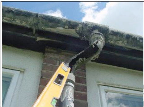
Asbestos gutters and downpipes in poor condition
