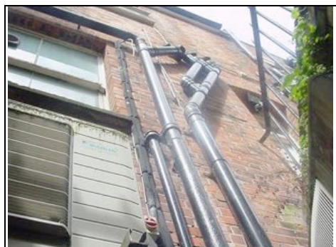
Soil and vent pipes at high level
