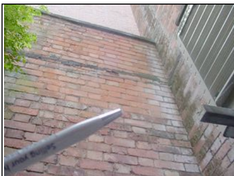
Rear elevation pattern staining and lichens
